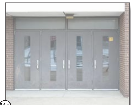
11C HOLLOW METAL DOORS & HOLLOW METAL FRAME
