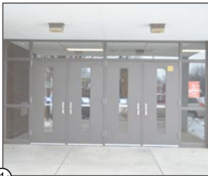
11J HOLLOW METAL DOORS & HOLLOW METAL FRAME
