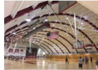
Field House Lighting
