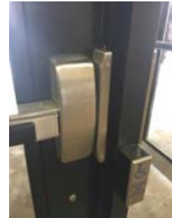
Keyless Entry Electric Strike
