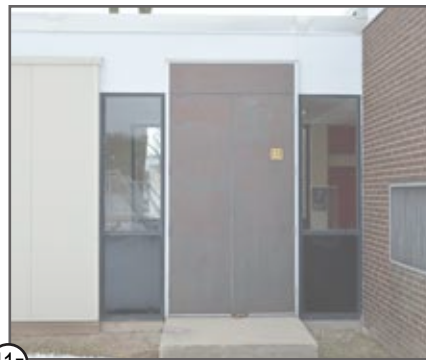
11F HOLLOW METAL DOORS & ALUMINUM FRAME
