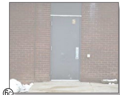
6C HOLLOW METAL DOOR & HOLLOW METAL FRAME
