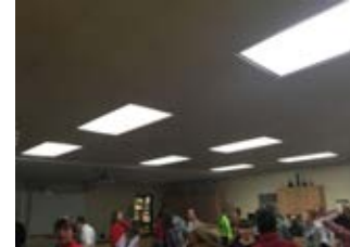
Typical Classroom Lighting
